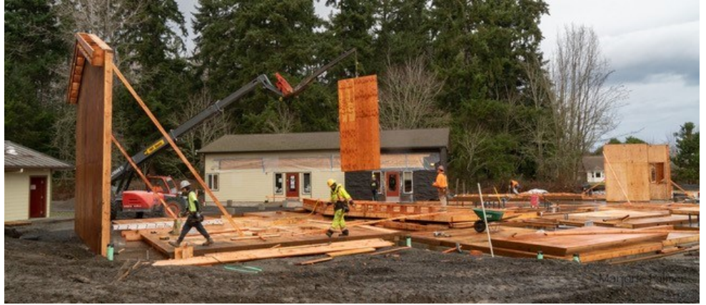
Construction of the new River Center in January 2021
